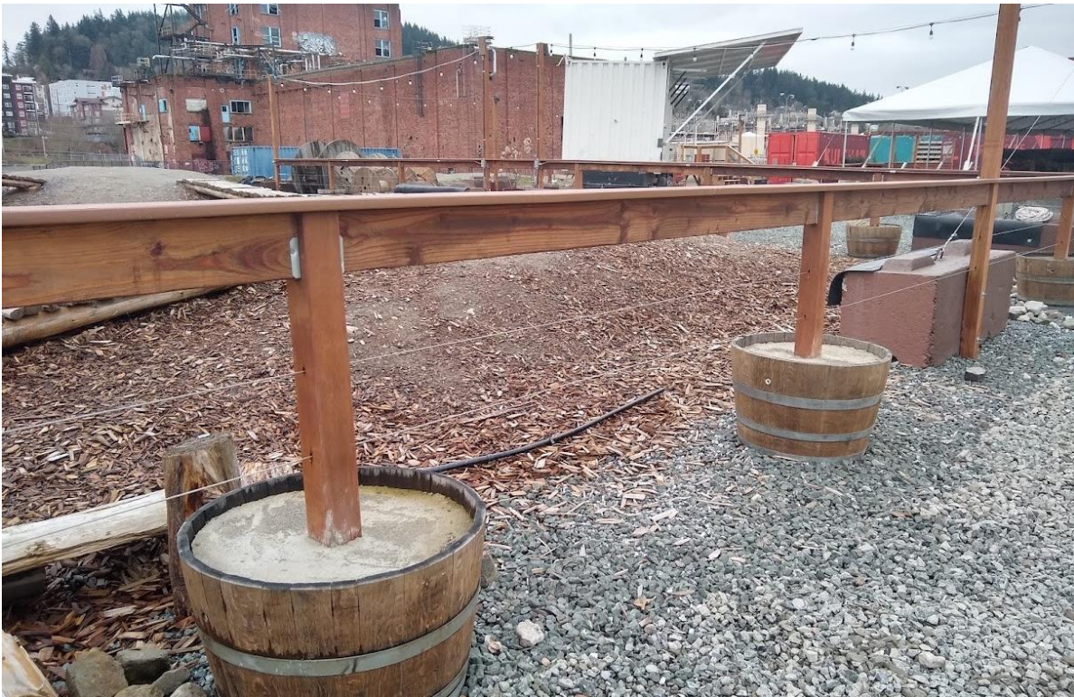
Cement-filled half barrels as temporary post stabilization
