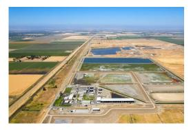
Plant upgrade: From 2013-2018, the Wastewater Treatment Plant was upgraded in order to meet State and Federal regulatory discharge requirements. The upgrade was accomplished in two phases: The Rehabilitation and Replacement (R&R) Phase and the Secondary and Tertiary Improvements (STI) Phase. The planning for upgrading local wastewater facilities began in 2001 when the Central Valley Regional Water Quality Control Board initiated new water discharge limits.
