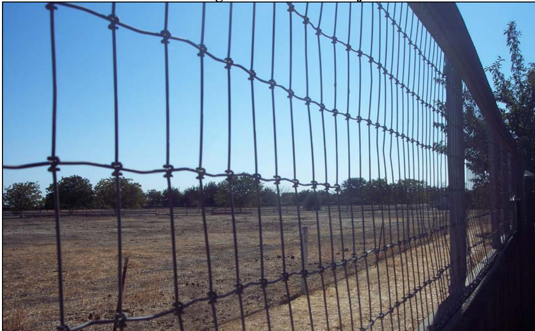
Figure 4.7-1 View Looking East across the Project Site
