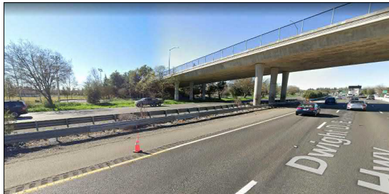
VIEW LOOKING SOUTHWEST FROM I-80 HWY. 08
