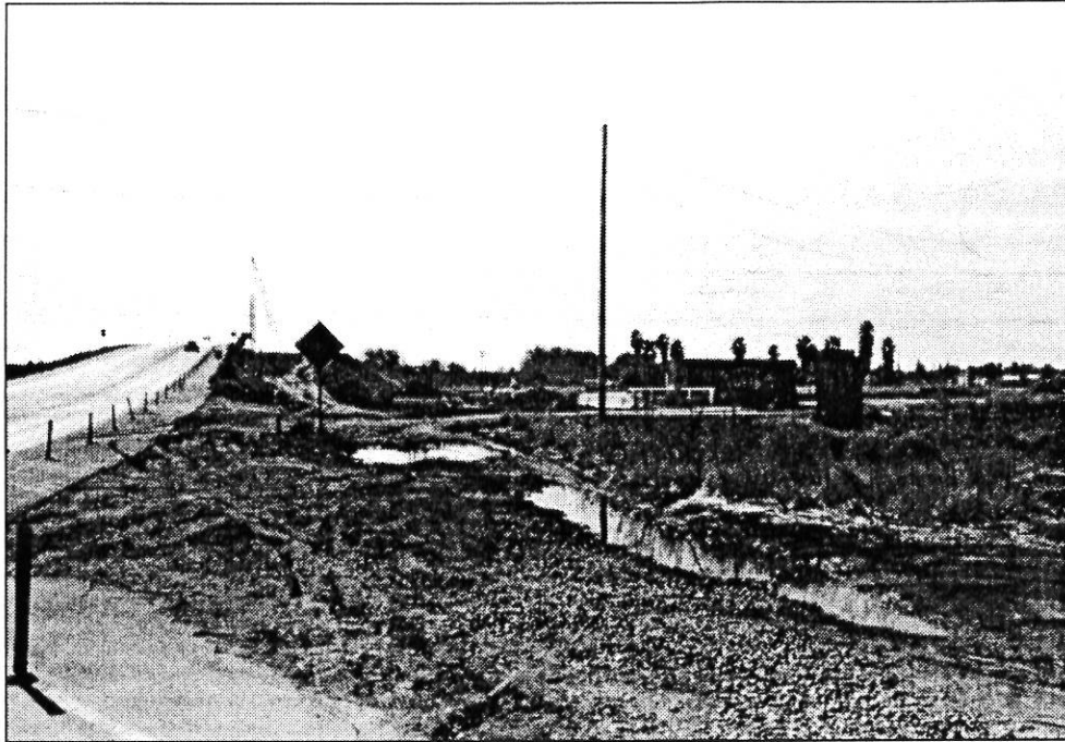
View of Under Second Street Site Facing South
