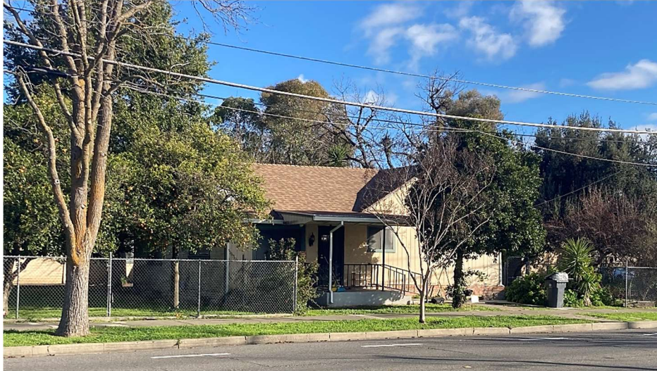
Partial view of west façade, facing northeast. Detached garage is visible in the left background. Source: ESA, 2024.
