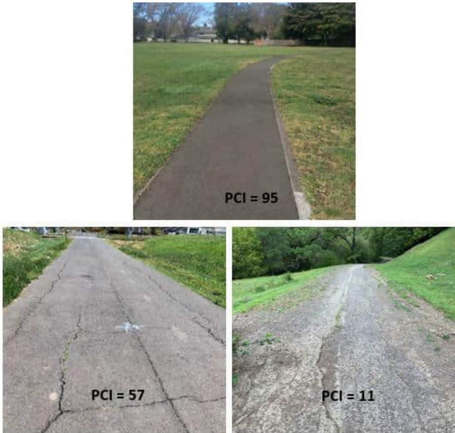
**Figure 2. Examples of Bike Paths with Different PCIs**
