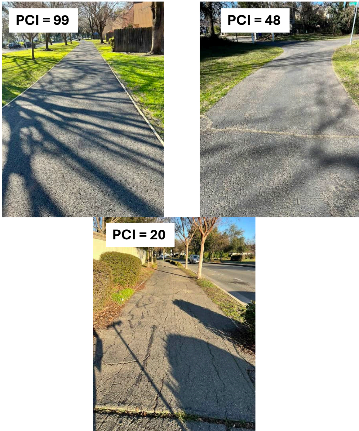
Figure 2. Examples of Bike Paths with Different PCIs
