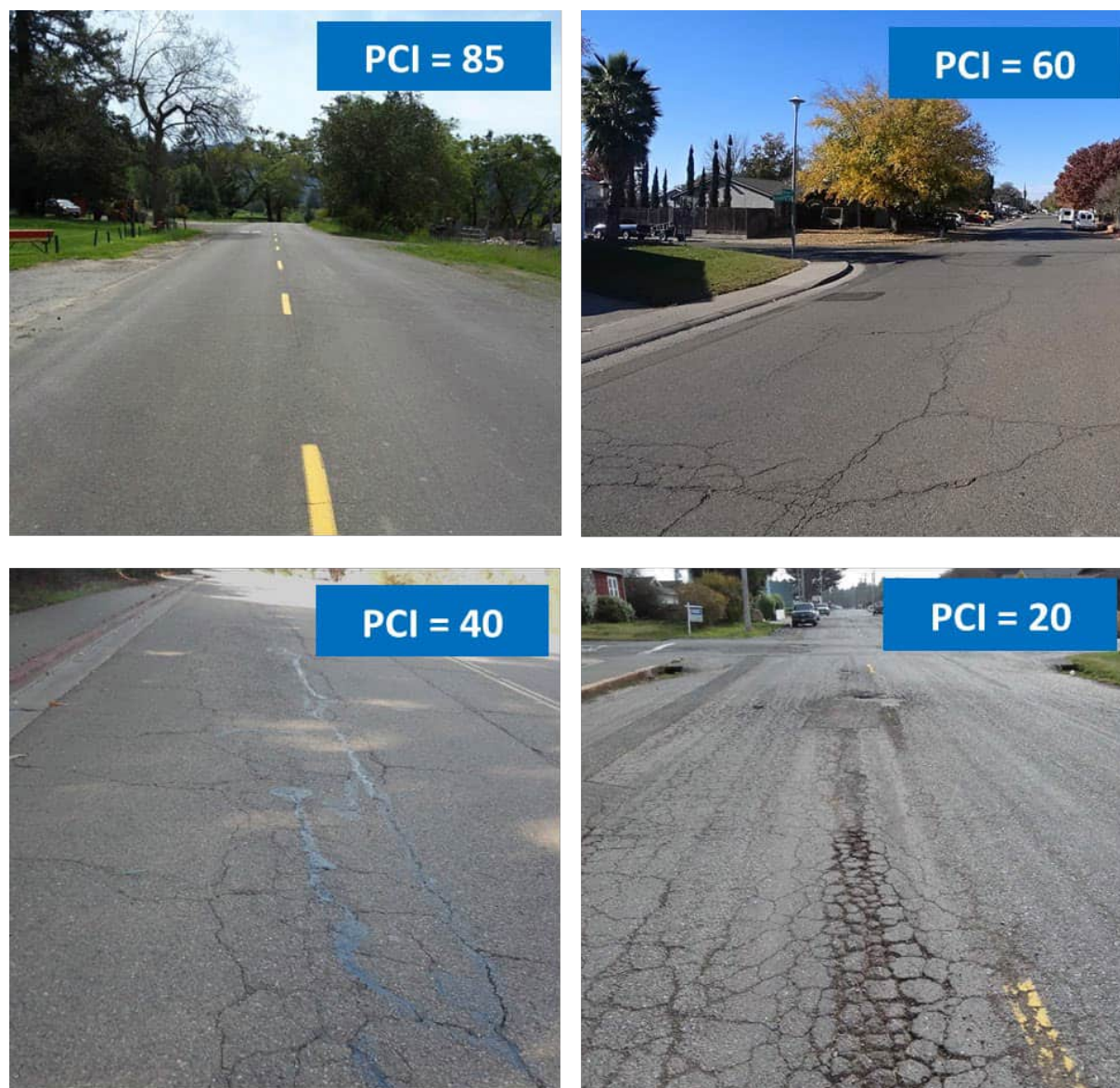
Figure 1. Examples of typical City Streets with Different PCIs
