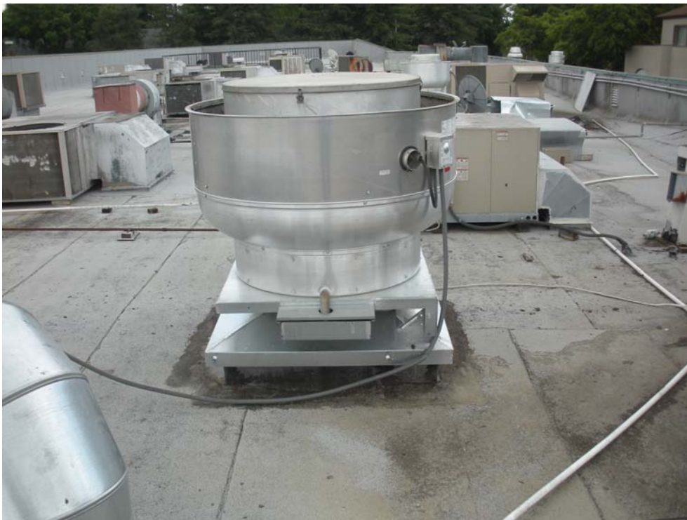
Example of one style of a grease collection tray on a kitchen exhaust fan.
