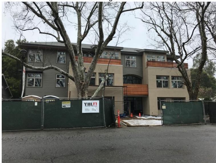
The Arbor Building 820 B Street
