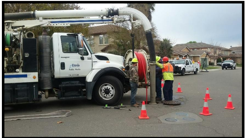
Storm Water Staff hydro-clean storm water mains as part of preventative maintenance.
