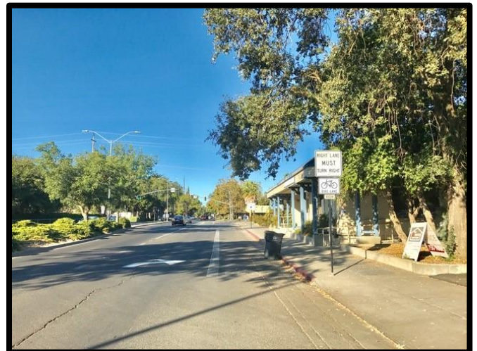
Lane improvements on Fifth Street with a dedicated right turn lane.
