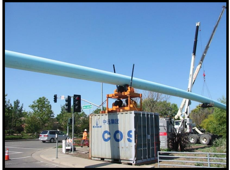
Surface water piping being lowered over John Jones Road before being installed underground.
