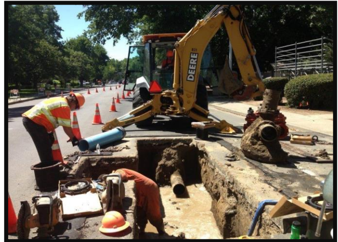
Water Division Staff repair a broken water main.
