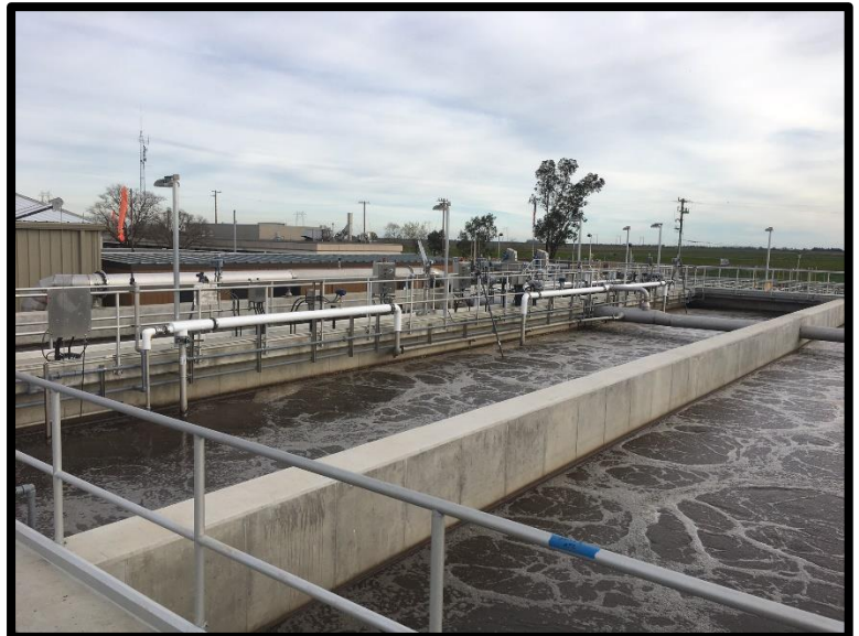
WWTP aeration basins at work.
