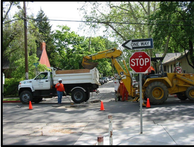
Collections Staff repair a 6" sewer main on Rice Lane.
