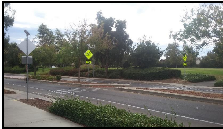
Rectangular Rapid Flashing Beacons (RRFBs) installed at Cowell and the Dave Pelz Bike Overcrossing.
