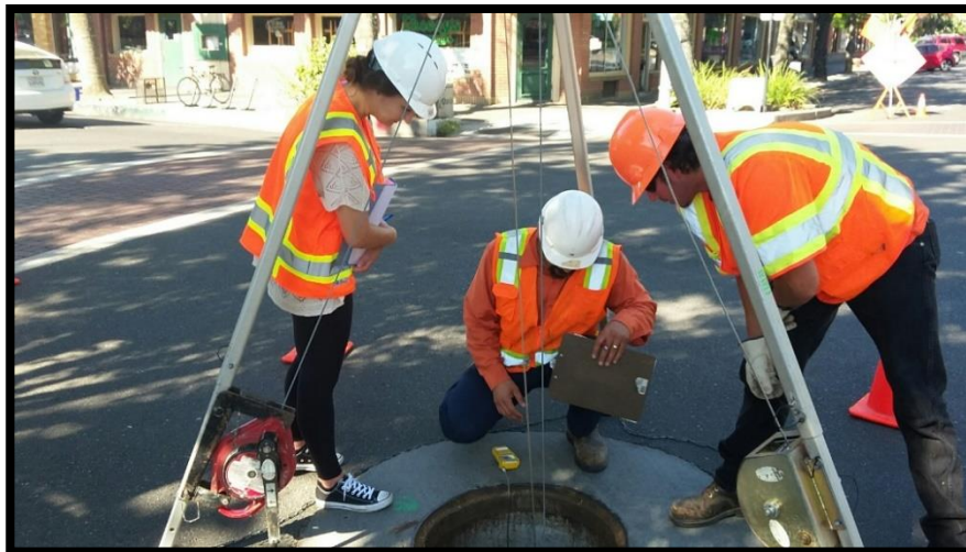
Staff take measurements as part of a survey of downtown drainage pipes.
