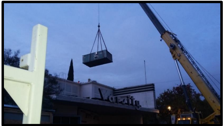
Varsity Theater receives a much-anticipated upgrade to their HVAC system. Staff delivered the unit in the early morning hours to minimize traffic disruption.
