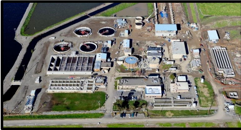
An aerial view of the Wastewater Treatment Plant as of March 2017.
