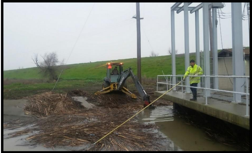
Staff removing storm debris surrounding a pump station.
