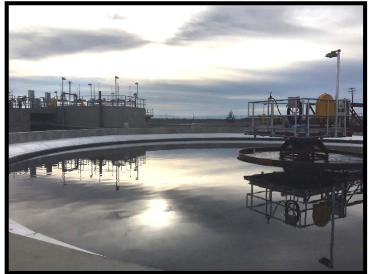
The Plant's secondary clarifier, which uses sedimentation to remove solids.
