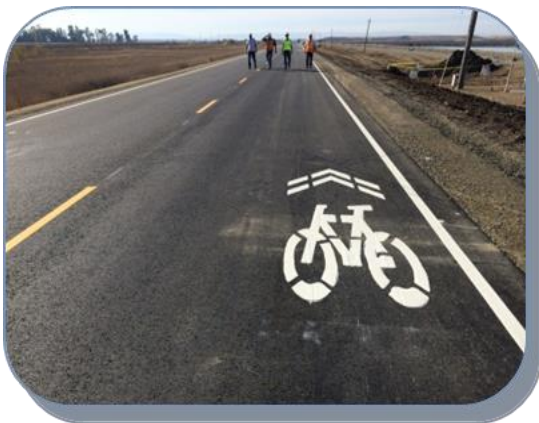
New Entrance Road to the WWTP
