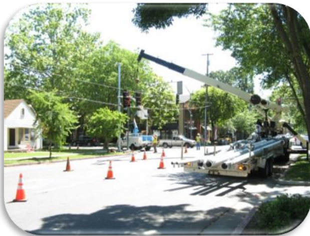
Fifth St. Project
