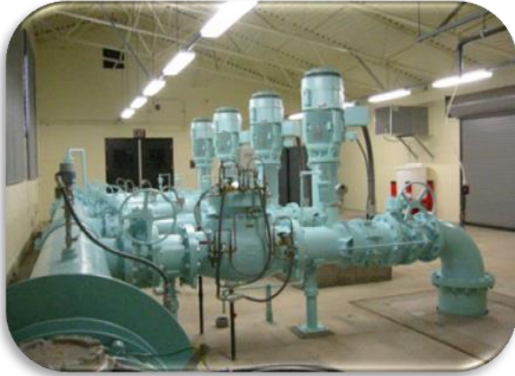
East Area Tank Pump Room
