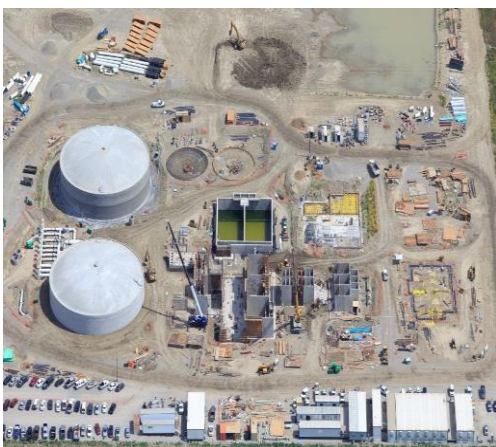
Davis Woodland Water Supply Project under construction April 2015
