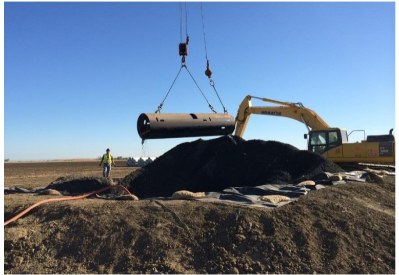
Sewer Trunk Line Sediment
