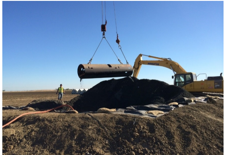
Sewer Trunk Line Sediment
