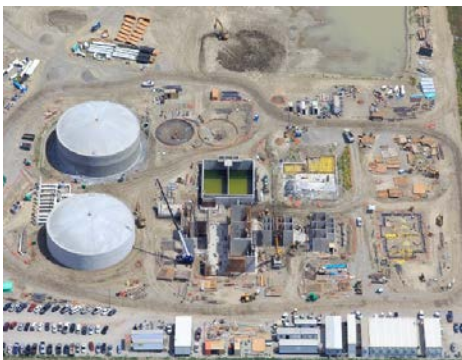
Davis Woodland Water Supply Project under construction April 2015
