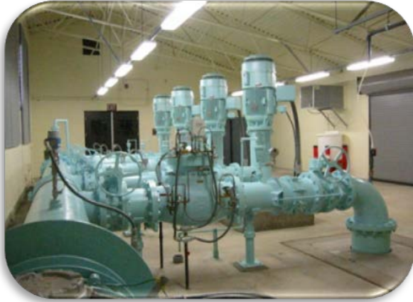
East Area Tank Pump Room
