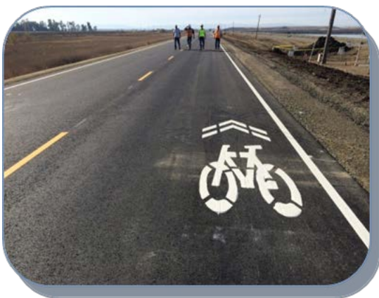
New Entrance Road to the WWTP
