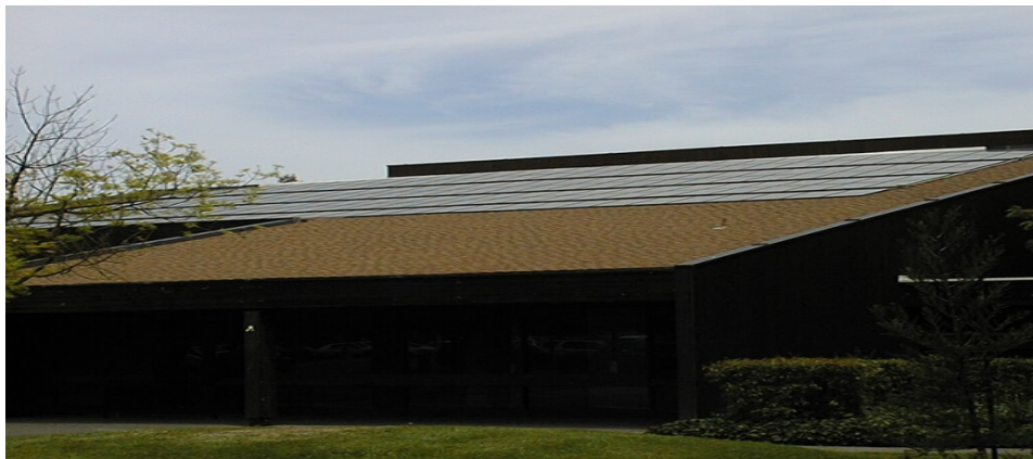
16.9 KW Photovoltaic System on the Veterans Memorial Center has produced electric power since July 2003
