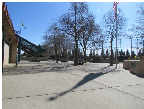
CDBG Funding used to make significant repairs to failing concrete pathways in the Playfields Park Complex, addressing public accessibility and safety.
