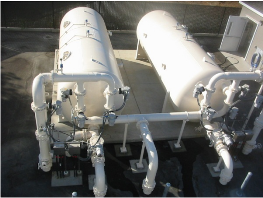
Manganese Filter Tanks
