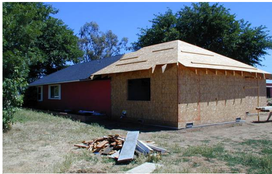
CDBG Funding used to expand Farmhouse facility which transitions mentally ill adults into the community
