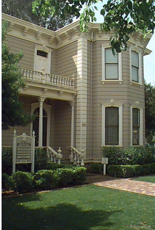
Hunt Boyer Mansion located at 604 2 nd street.
