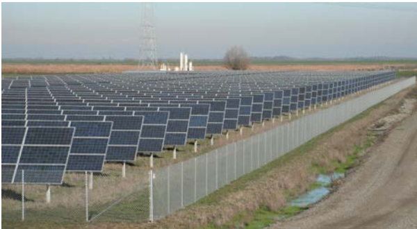
Solar Panels at the Wastewater Treatment Plant
