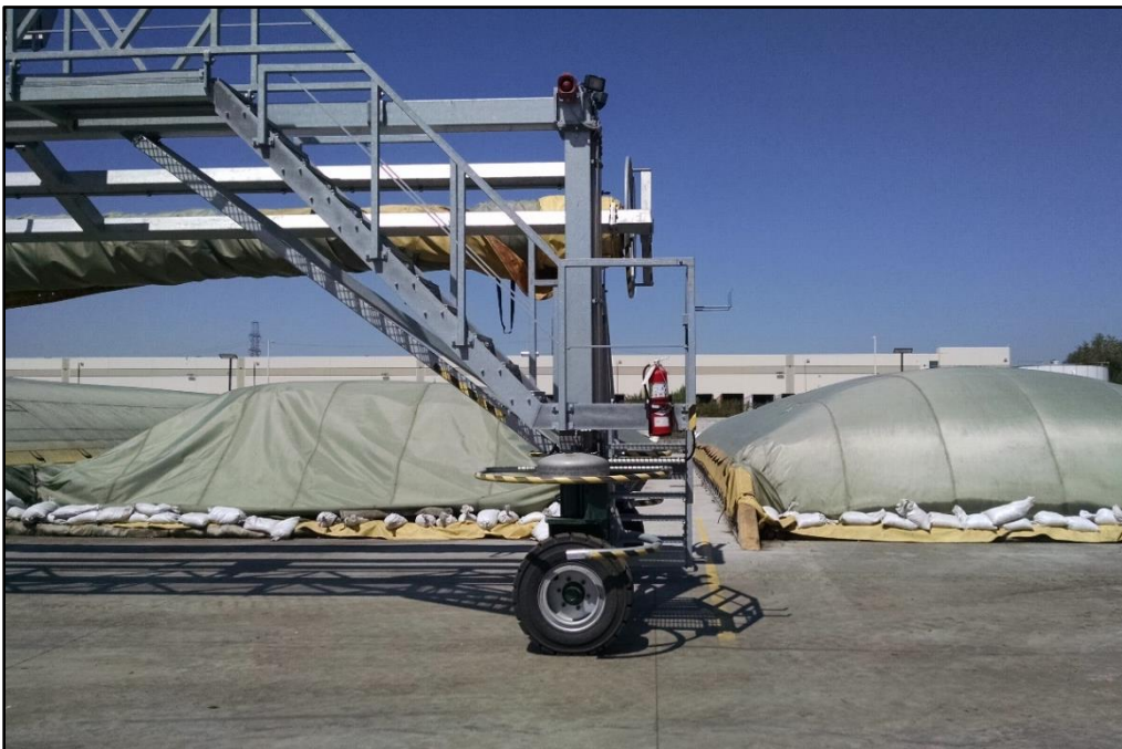
Figure 6.12 GORE® Composting Facility Compost Piles
