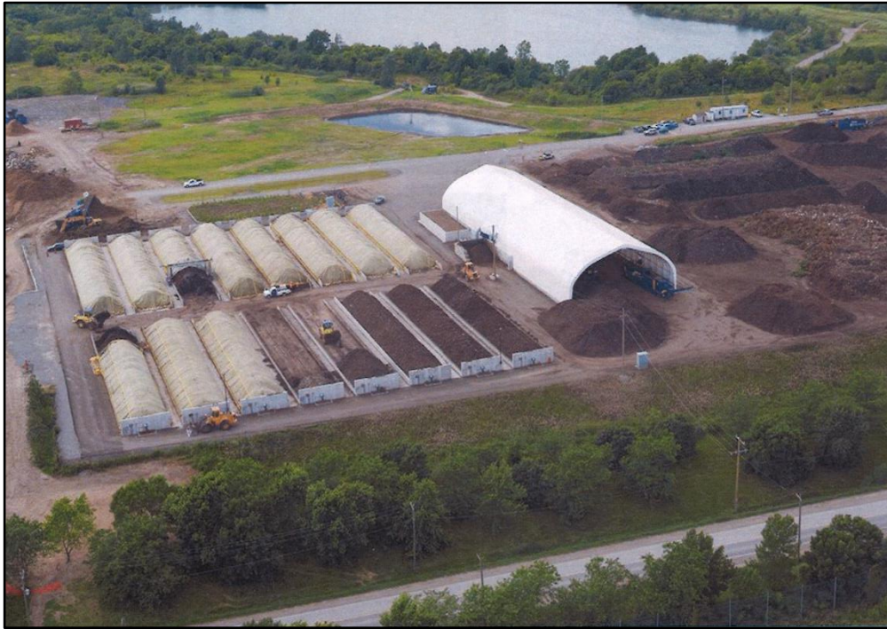
Figure 6.11 GORE® Composting Facility Aerial (Source: Sustainable Generation)
