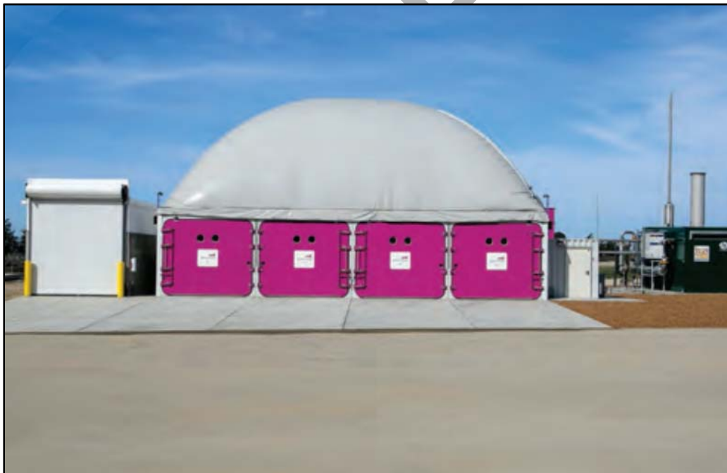
Figure 6.12 SMARTFerm System at Monterey Regional Waste Management District (Source: SMARTFerm)
