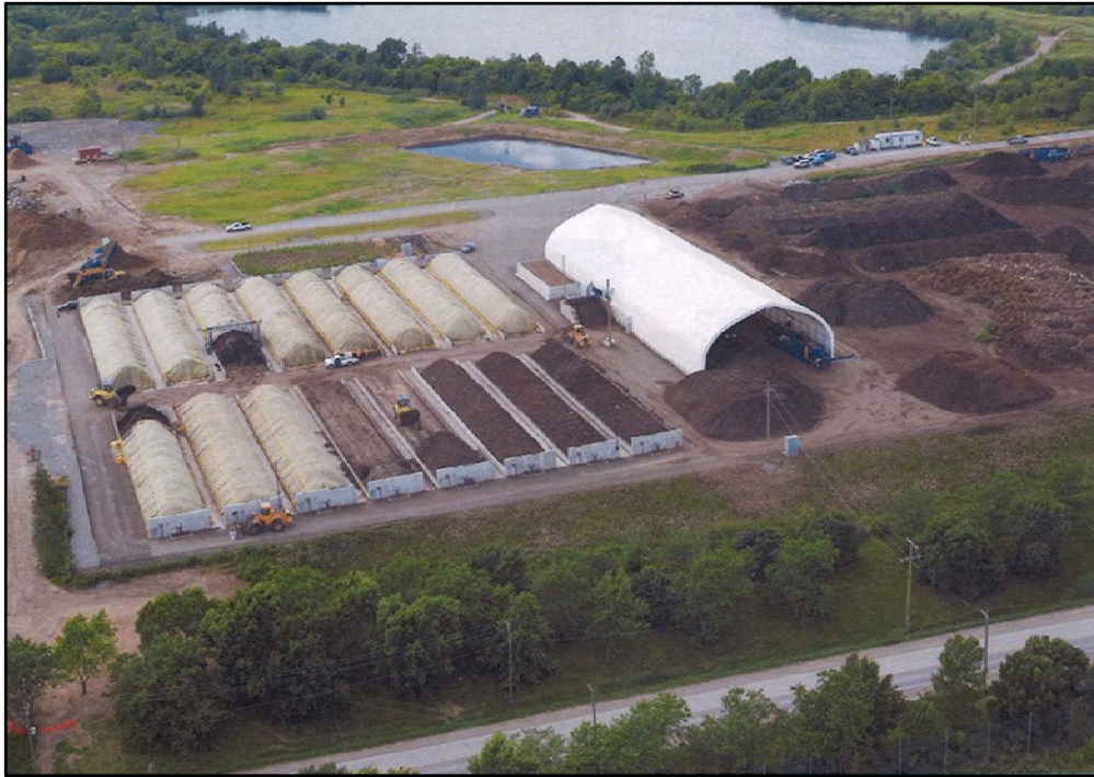
Figure 6.10 GORE® Composting Facility Aerial (Source: Sustainable Generation)
