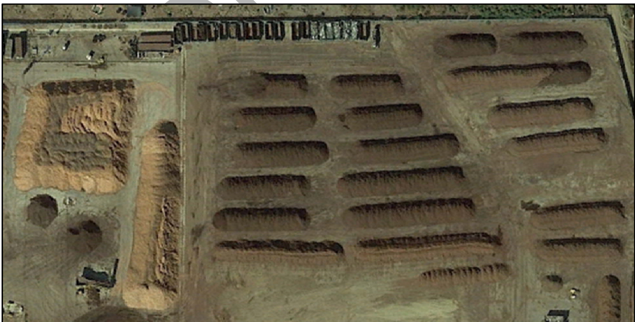
Figure 6.8 Example Static Pile Composting Facility Aerial (Source: Google Earth)
