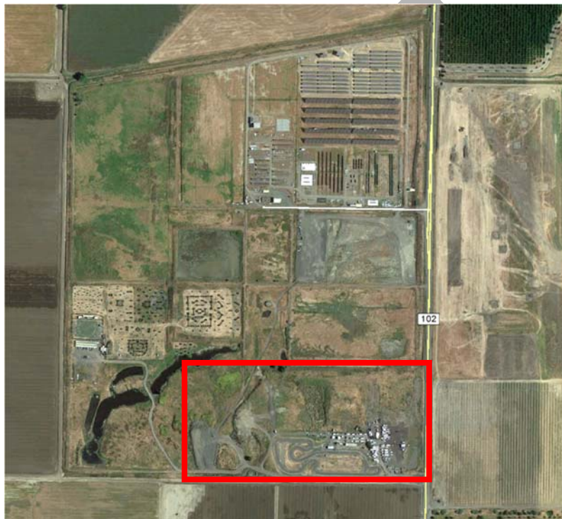
Figure 6.4 Old City of Davis Landfill Available Land (Source: Google Earth)
