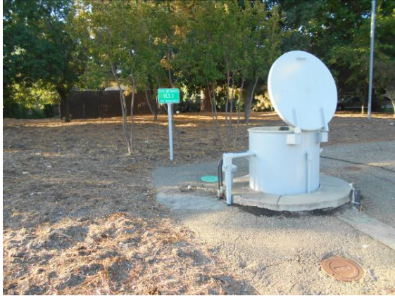
Access to Station Dry Pit
