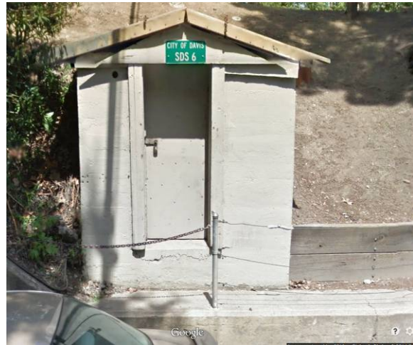
Pump Station Building
