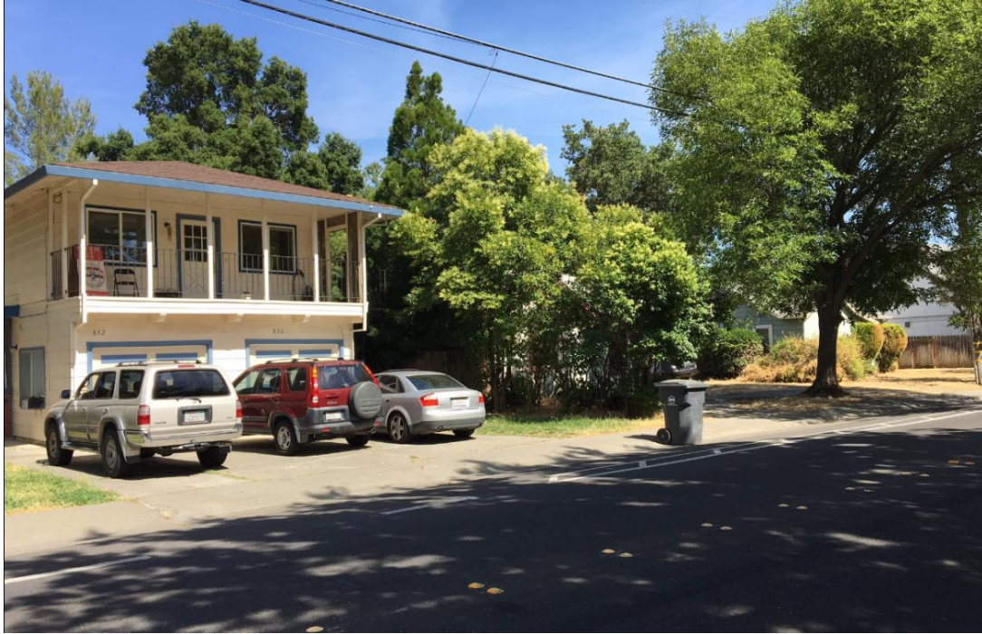
Adjacent 2-story Duplex Located North of 822 B Street
