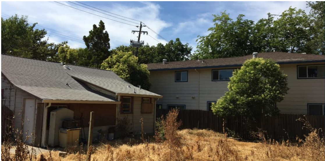
822 B Street Rear Yard View of Adjacent Duplex
