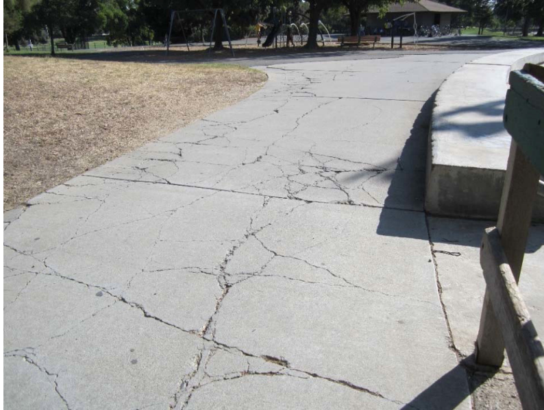
The pedestrian pavements have damage requiring full depth replacement.
