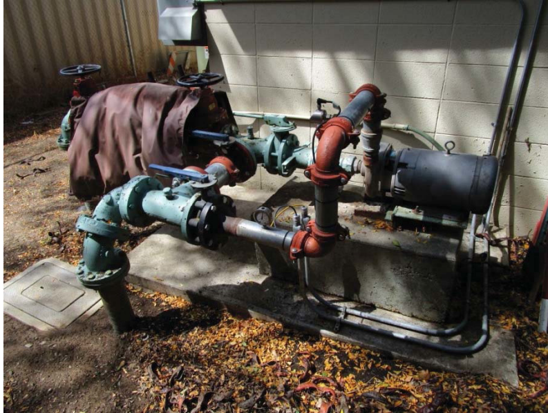
The Maintenance Building backflow preventer is at the end of its expected useful life.
