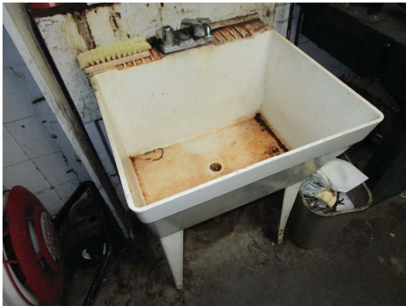
The Maintenance Building plumbing system and plumbing fixtures are at the end of their expected useful lives.
