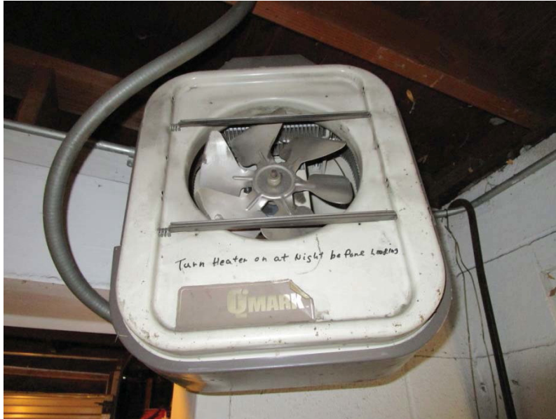
The Maintenance Building electric unit heater as well as all HVAC equipment are at the end of their industry standard expected useful life.
