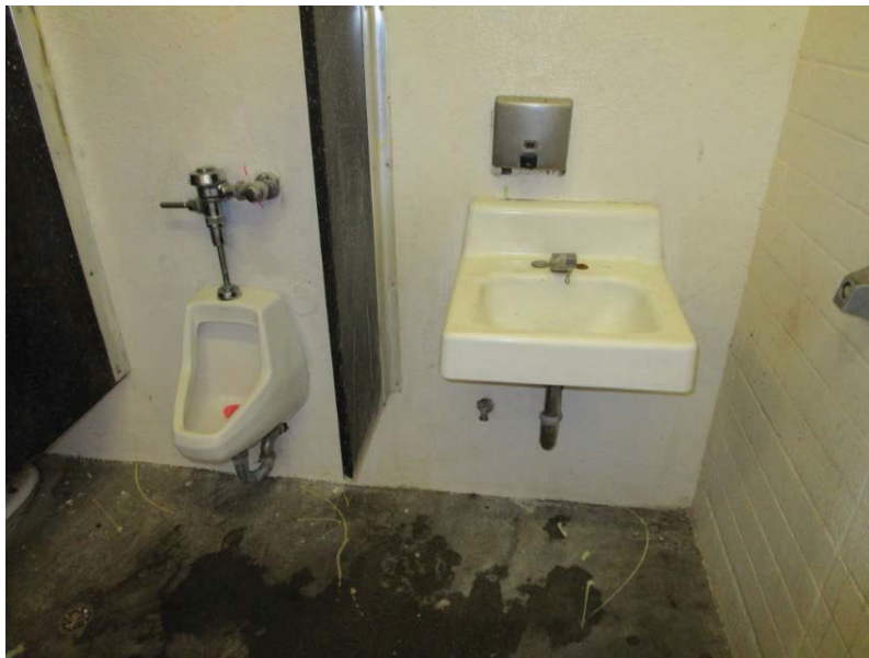
The restroom plumbing system and plumbing fixtures are at the end of their expected useful lives.
