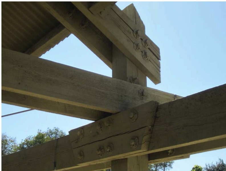
The wood picnic shelter has cracking throughout, requiring replacement.
