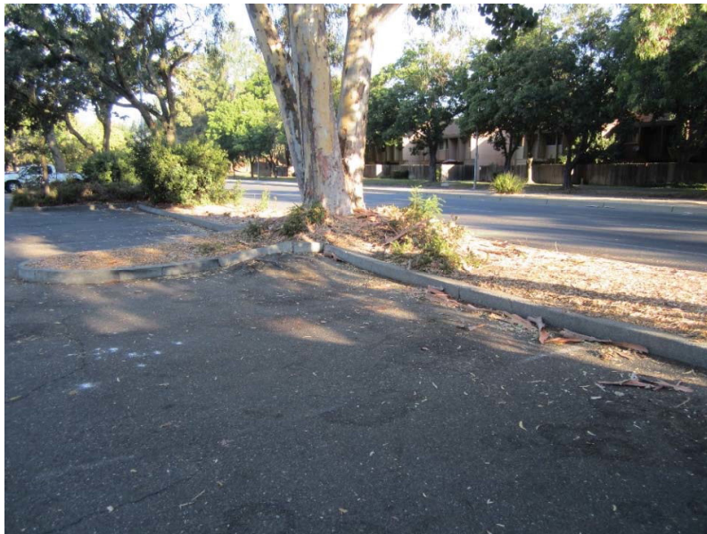
The parking lot pavement has structural damage (example – tree roots) requiring full depth replacement.
