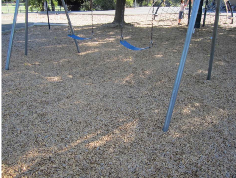
The playground surfacing needs additional material due to ruts beneath equipment.
