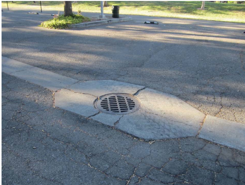
The drainage gutters and curbs in the parking lot have damage requiring replacement.
