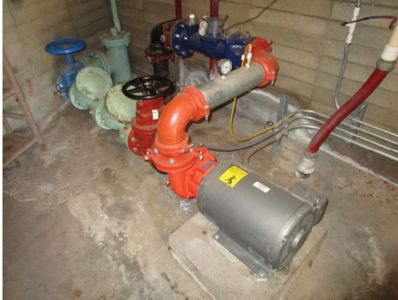
The restroom building backflow preventer is at the end of its expected useful life.
