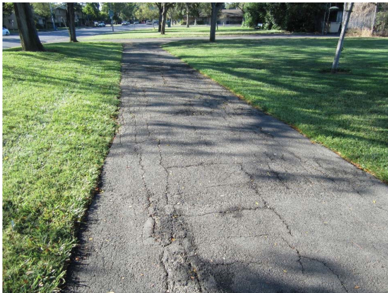
The bike paths have damage requiring repairs or replacement.
