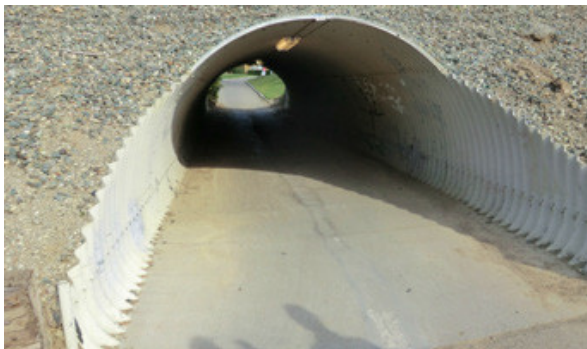
EXISTING H STREET TUNNEL
