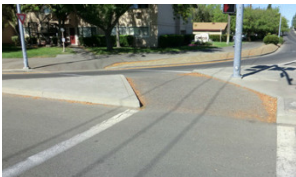
J STREET PEDESTRIAN ROUTE THROUGH CHANNELISED RIGHT TURN
