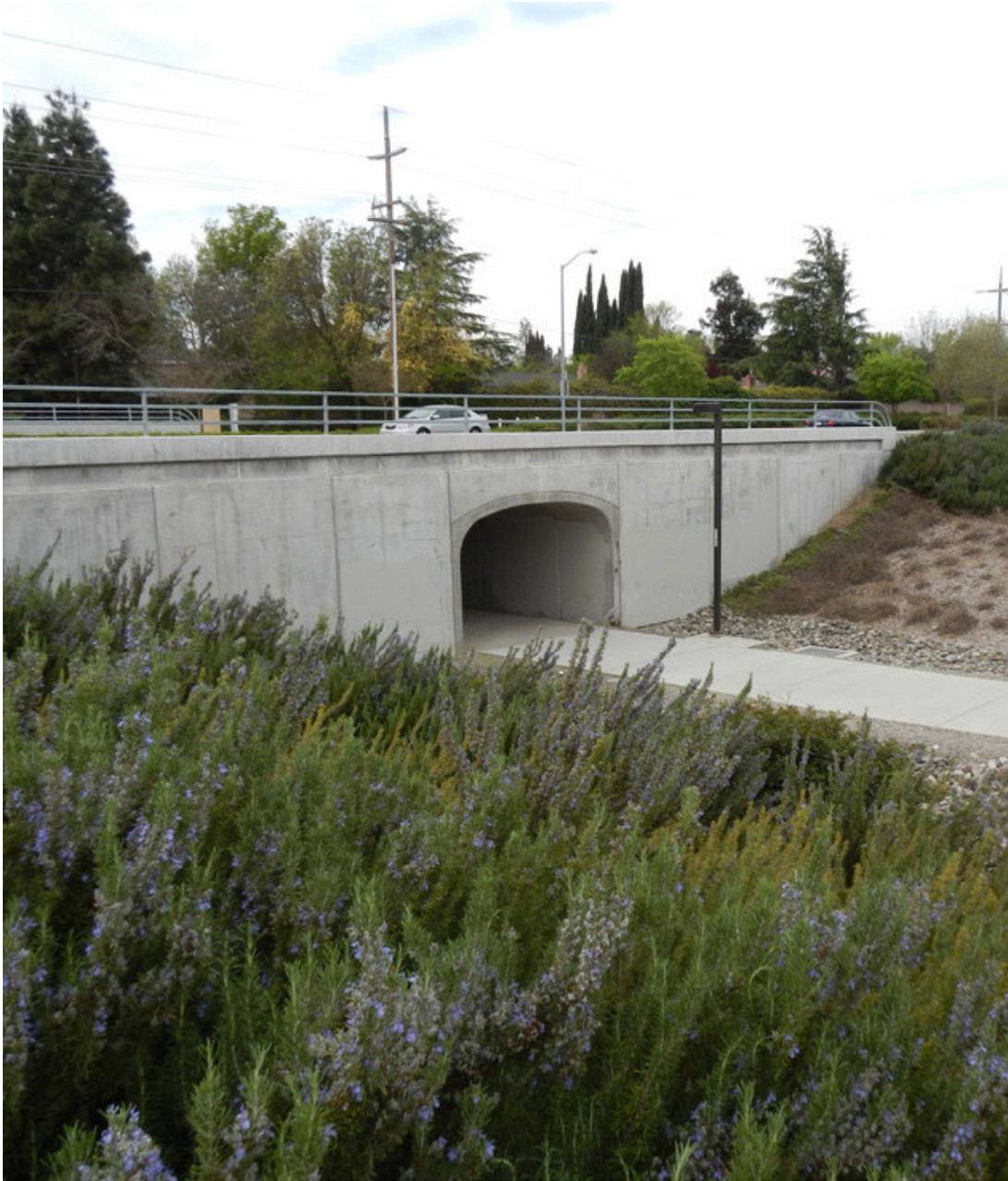
ALHAMBRA SHARED-USE TUNNEL
