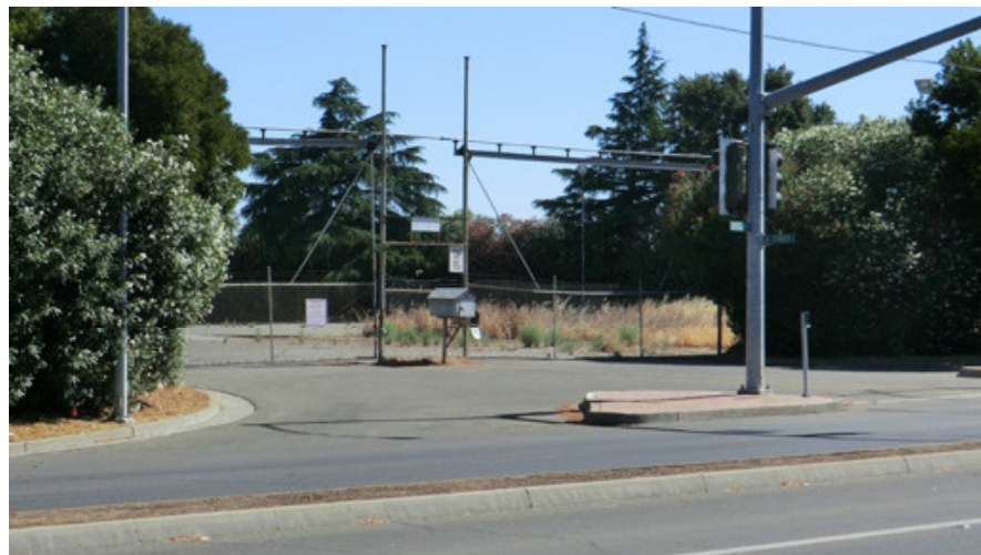
LOOKING NORTH AT J STREET AND COVELL BOULEVARD
