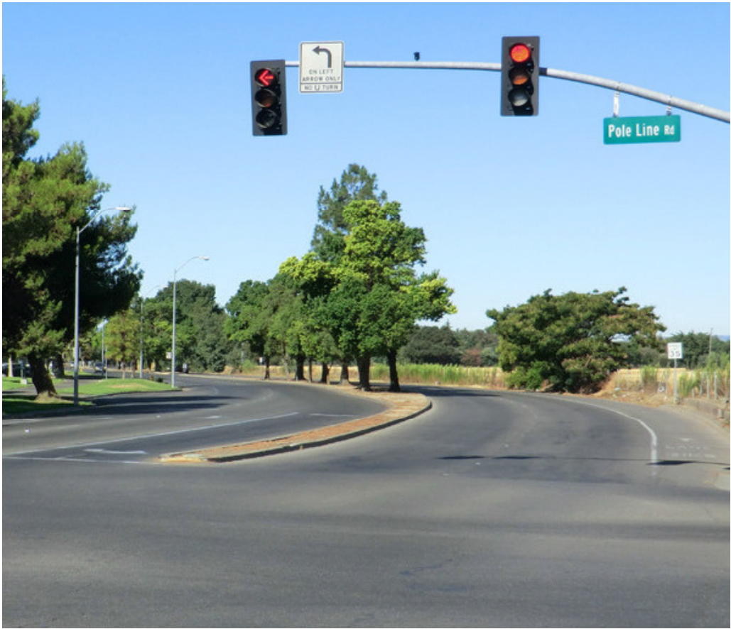
COVELL BOULEVARD LOOKING WEST AT POLE LINE ROAD
