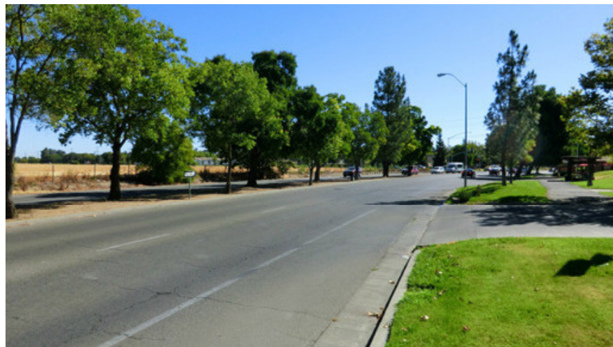
COVELL BOULEVARD AT OAK TREE PLAZA LOOKING EAST
