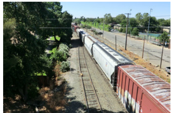
EXISTING RAILROAD TRACKS NEAR F STREET
