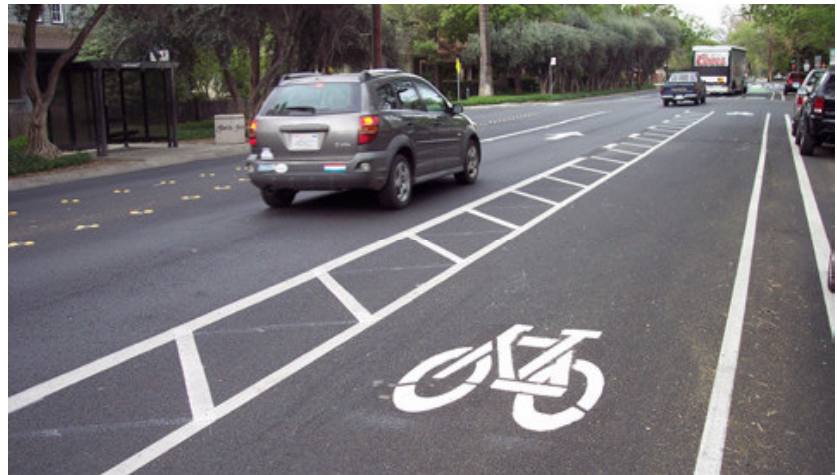
EXAMPLE OF A BUFFERED BICYCLE LANE 1 ST STREET IN DAVIS
