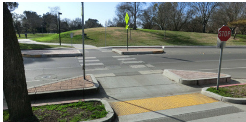
F STREET PEDESTRIAN CROSSING
