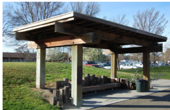
EXISTING BUS SHELTER NEAR POLE LINE ROAD AND COVELL BOULEVARD
