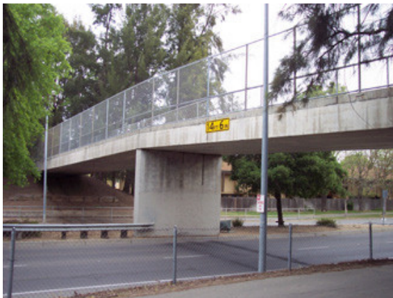
PEDESTRIAN BRIDGE WEST OF F STREET
