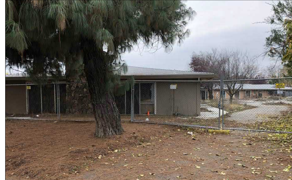
18 LOOKING WEST AT SITE FROM FRONT SETBACK
