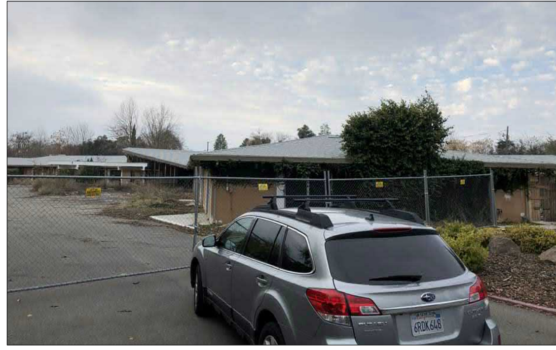
6 LOOKING WEST FROM DRIVEWAY
