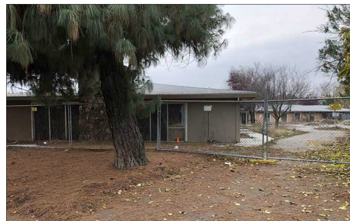
18 LOOKING WEST AT SITE FROM FRONT SETBACK
