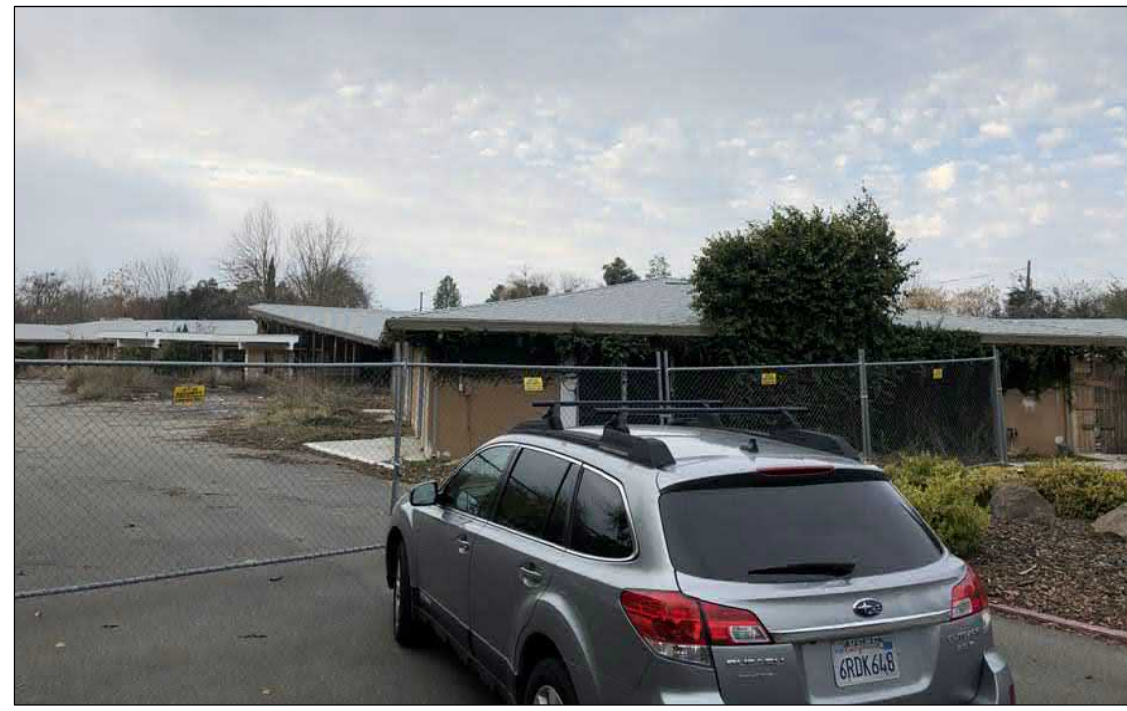
6 LOOKING WEST FROM DRIVEWAY
