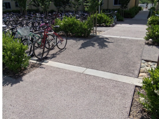
Pervious pavement in a bike parking area allows for a solid surface while still allowing infiltration.
