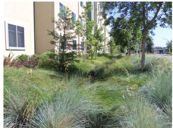
Vegetated swale outside of Tercero II Housing, UC Davis campus, promotes stormwater filtration and infiltration.
