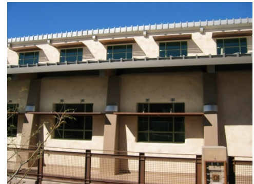
Figure 4-10 Example of Light Shelves in Commercial Building
