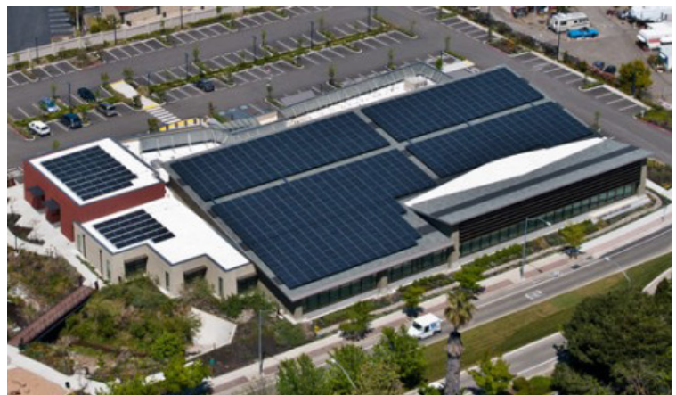
(Photo Courtesy of Sun Light & Power)
