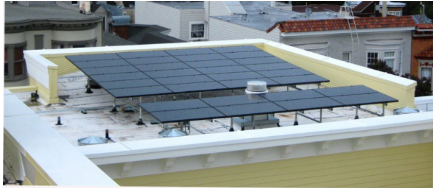
(Photo Courtesy of Sun Light & Power)
