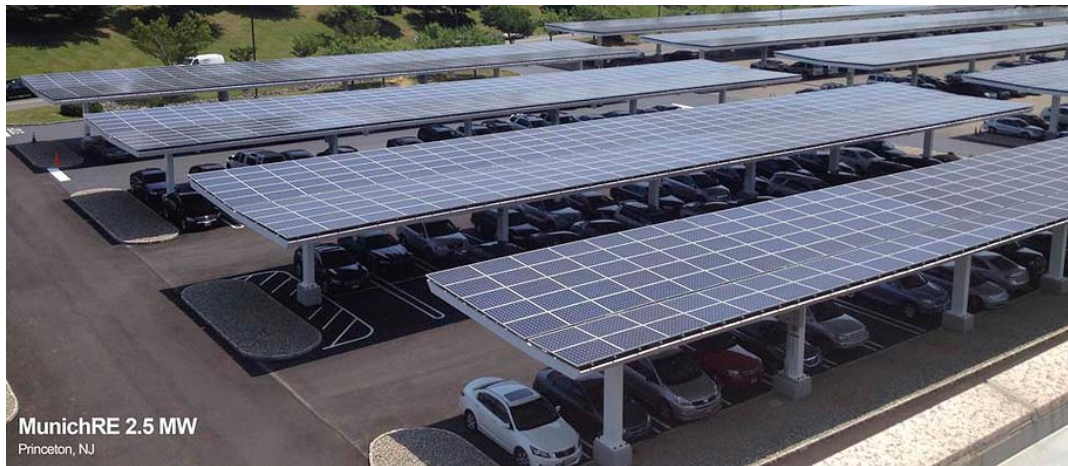
Figure 4-16 Parking Lot Shading PV System Installations
