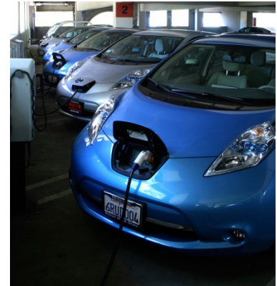
Providing dedicated parking spaces and infrastructure for electric vehicles to charge is essential sustainability infrastructure.
