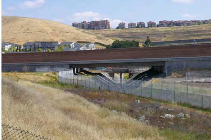
Failed mitigation: Never maintained.
