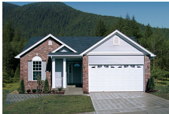
Garage and driveway are too prominent. Porch and columns are not balanced with other massing. Material shifts are forced.
