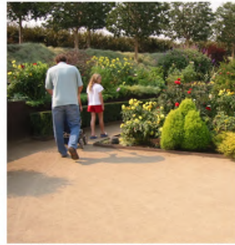
Stabilized decomposed granite paving
