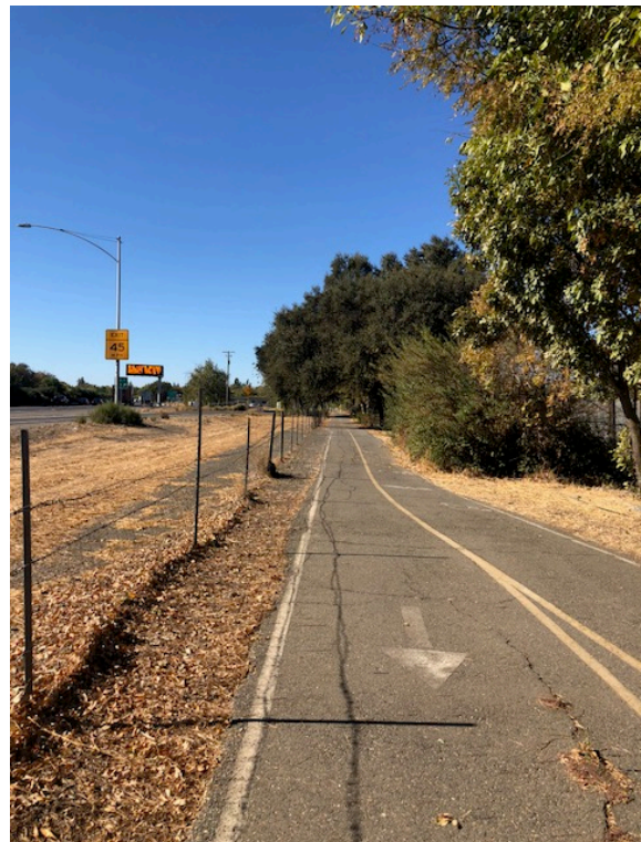
Photo 4: View of existing bike path looking west.
