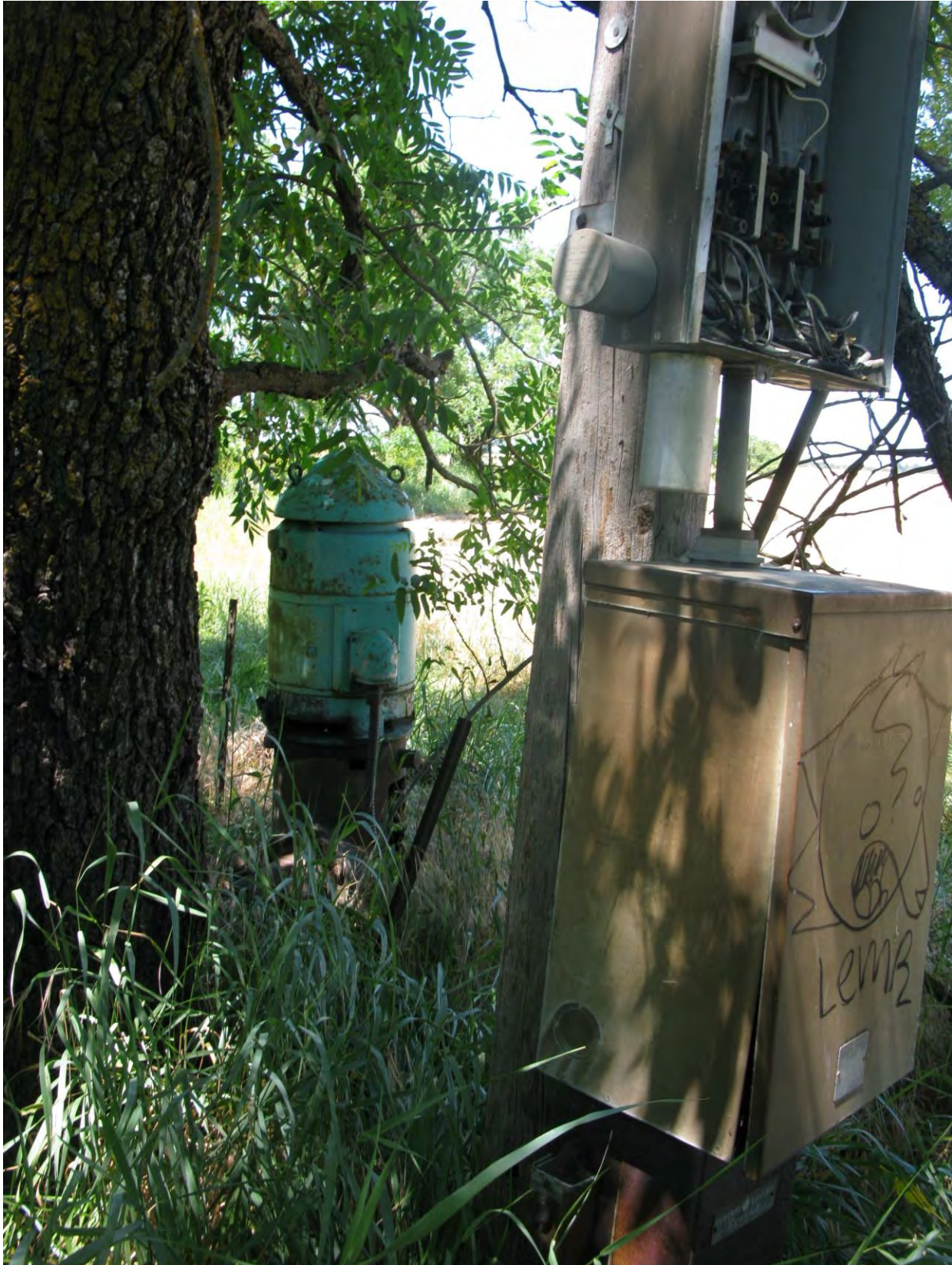
D) View of the above ground pump and electrical service drop/panel, looking west. 6-12-17. Acc.20170615fr65
