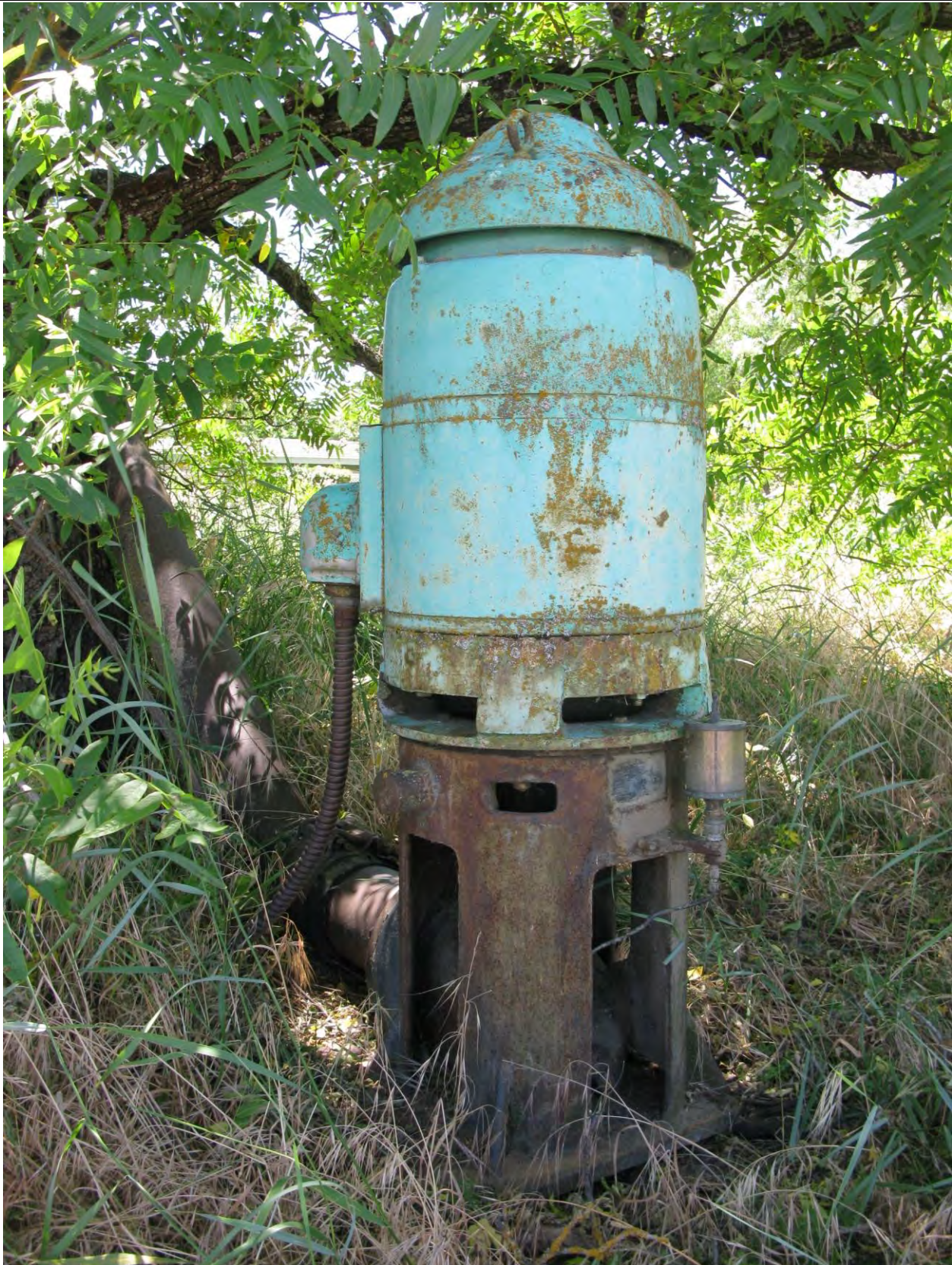
A) View of the above ground pump, older pump base, looking southwest. 6-12-17. Acc.20170615fr60
