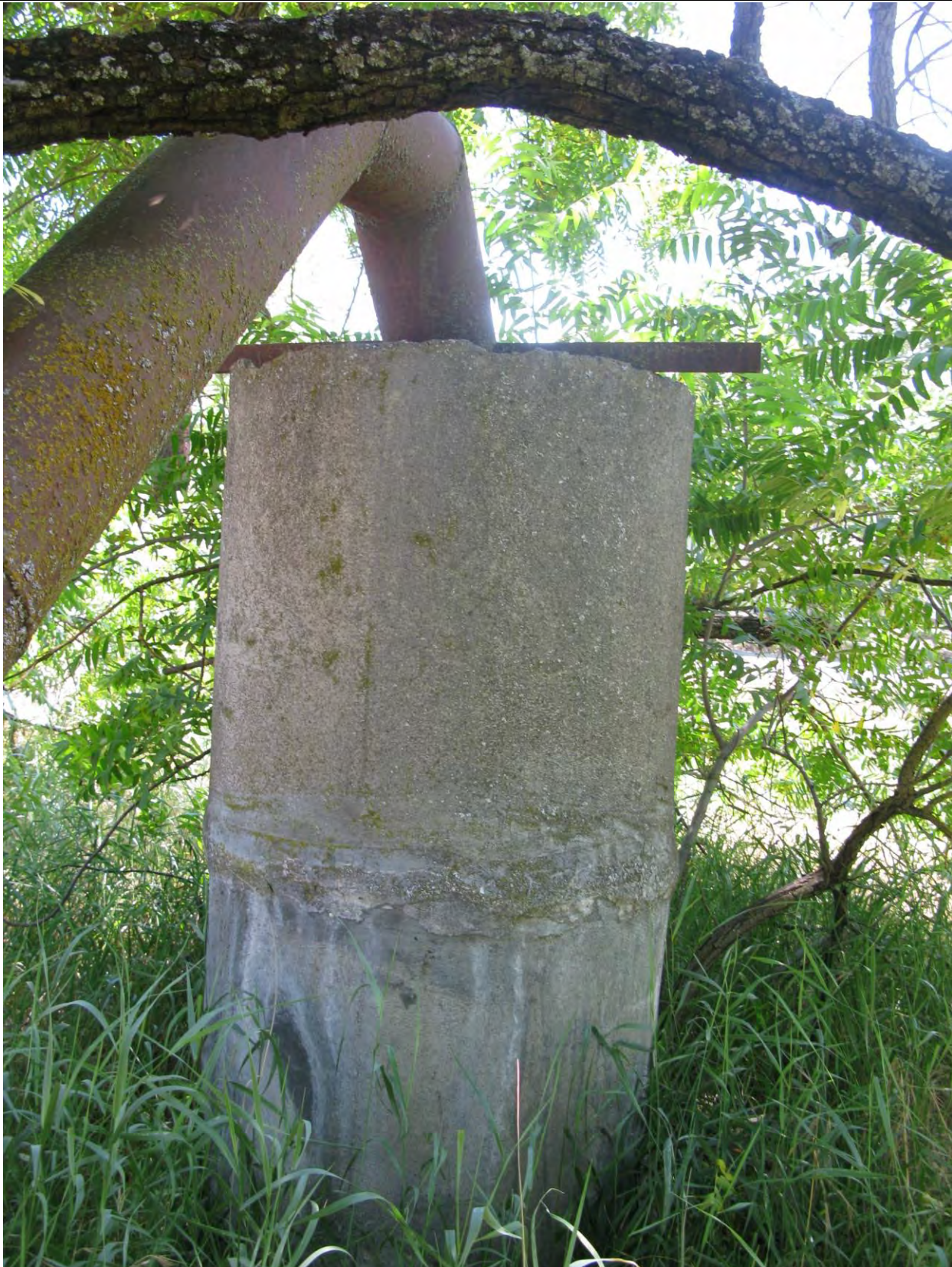
C) View of the southern portion of the pipe, stand pipe, looking southeast. 6-12-17. Acc.20170615fr64
