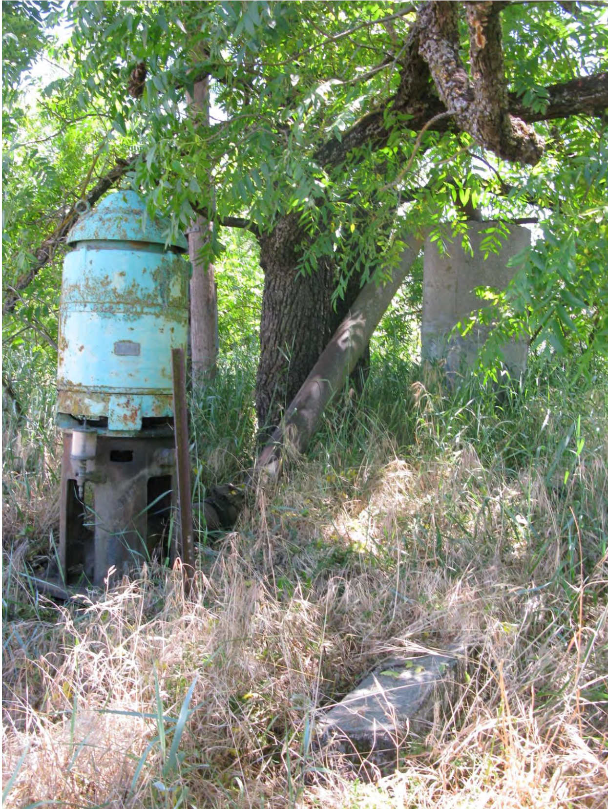
B) View of the above ground pump (left), pipe (center), stand pipe (right) looking southeast. 6-12-17. Acc.20170615fr62
