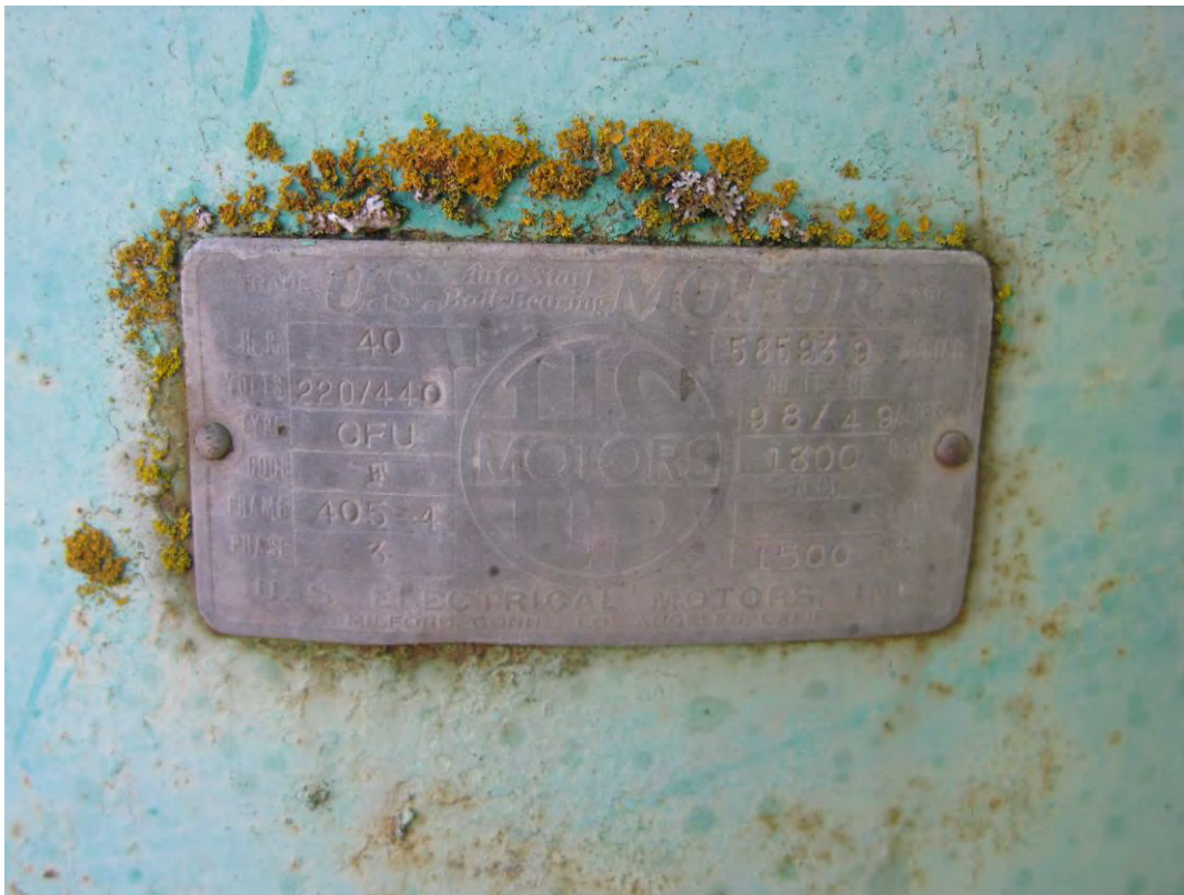
H) View of the plate located on the above ground pump. 6-12-17. Acc. #20170615fr63
