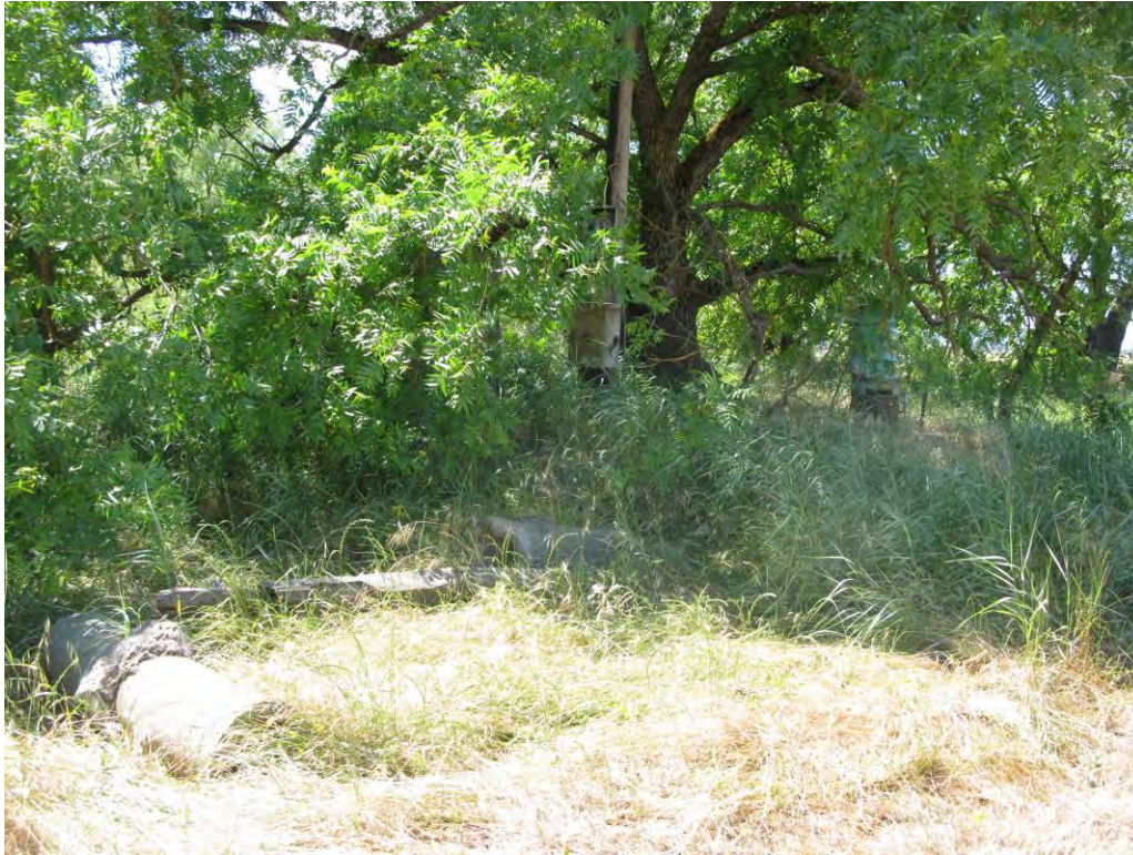
E) View of scattered concrete posts, above ground pump and electrical service drop/panel in background, looking south. 6-12-17. Acc. #20170615fr77
