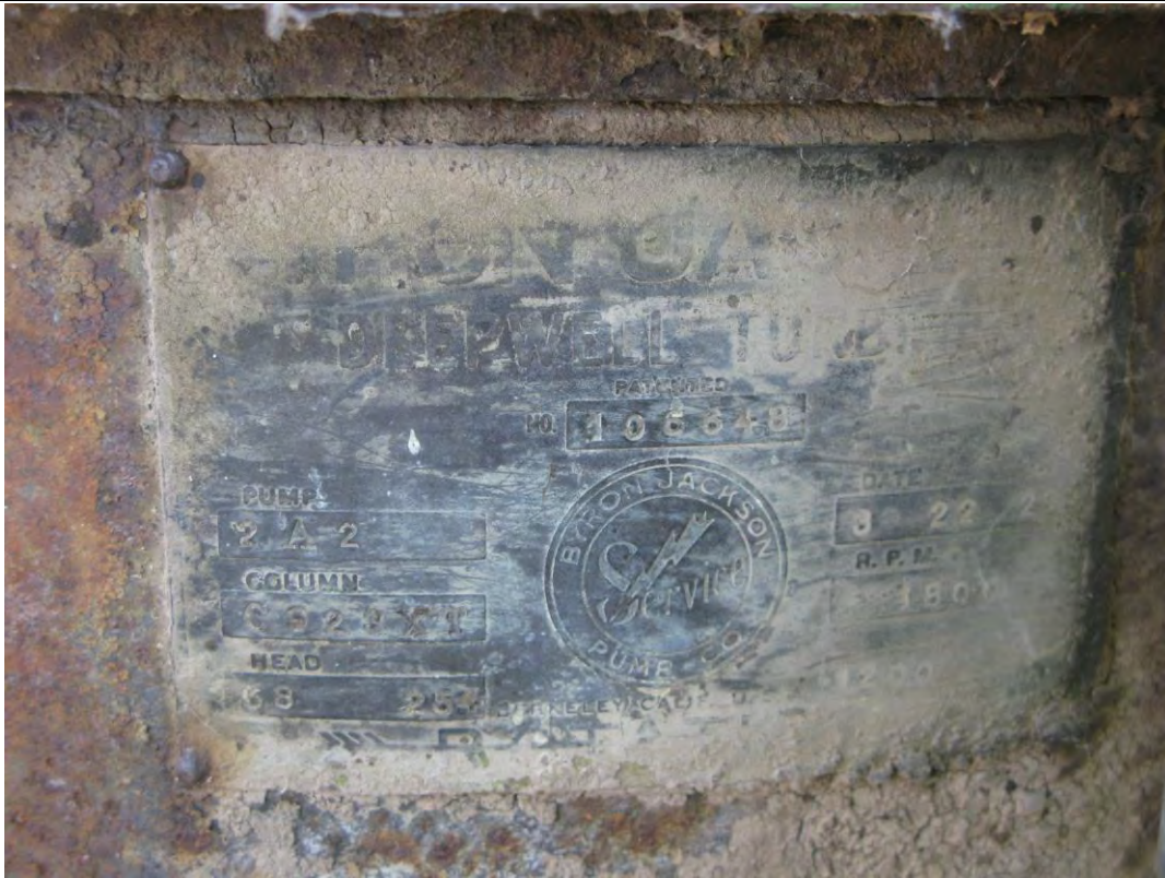
G) View of the plate located on the base of the above ground pump. 6-12-17. Acc. #20170615fr61
