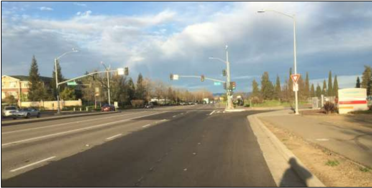
VIEW OF WEST COVELL BOULEVARD/RISLING COURT/SHASTA DRIVE SIGNALIZED INTERSECTION.
