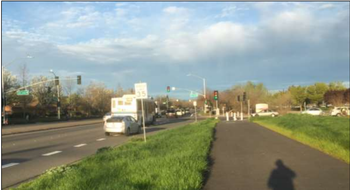
VIEW OF CLASS I SHARED-USE PATH ON NORTH SIDE OF WEST COVELL BOULEVARD EAST OF JOHN JONES ROAD
