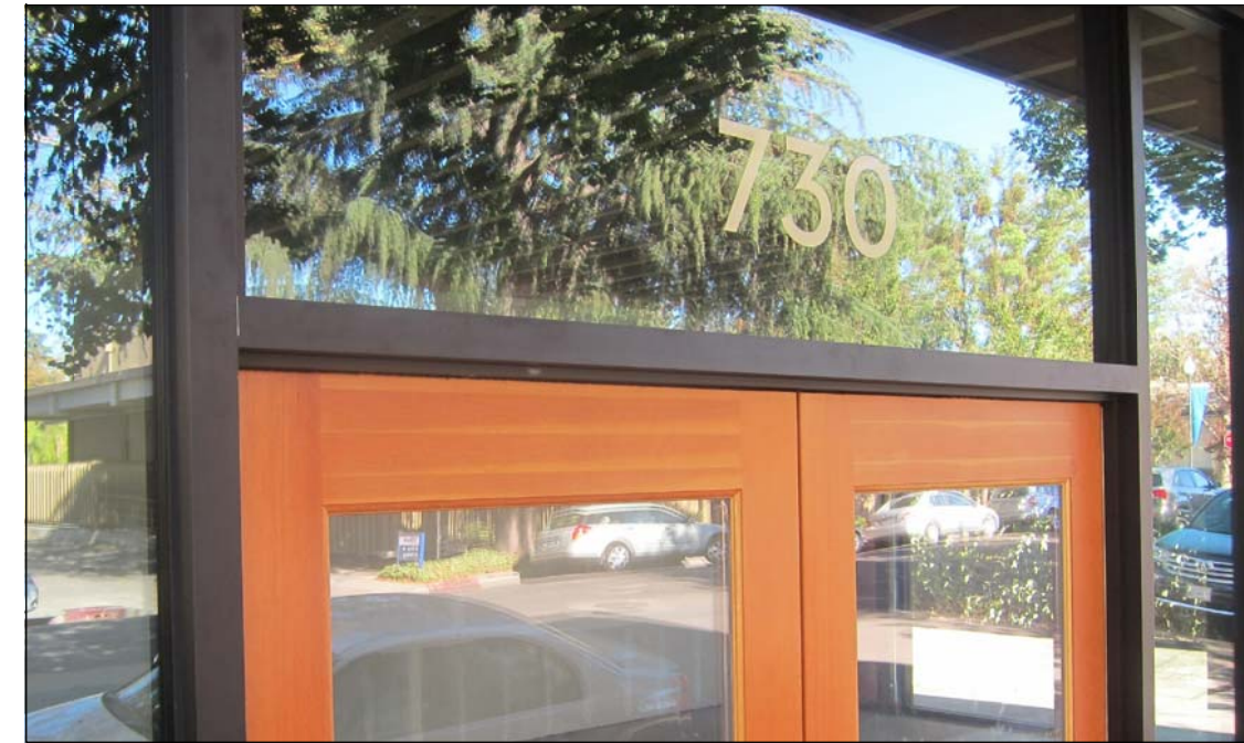
12 DARK BRONZE STOREFRONT GLAZING WITH CLEAR FINISH VGDF DOORS
