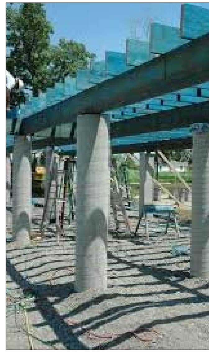
7 CONCRETE PIERS SUPPORTING TRELLIS
