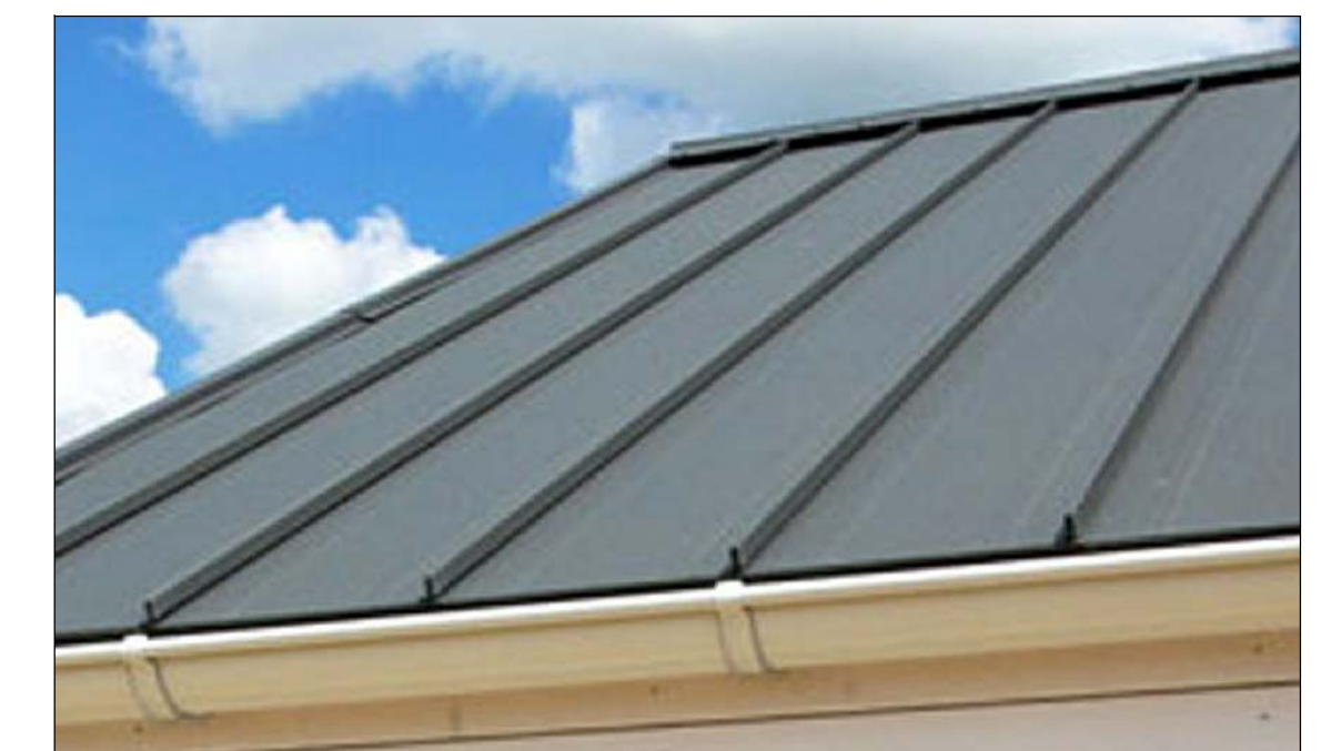
1 NATURAL ZINC STANDING SEAM METAL ROOF (ALTERNATE AT ENTRY)
