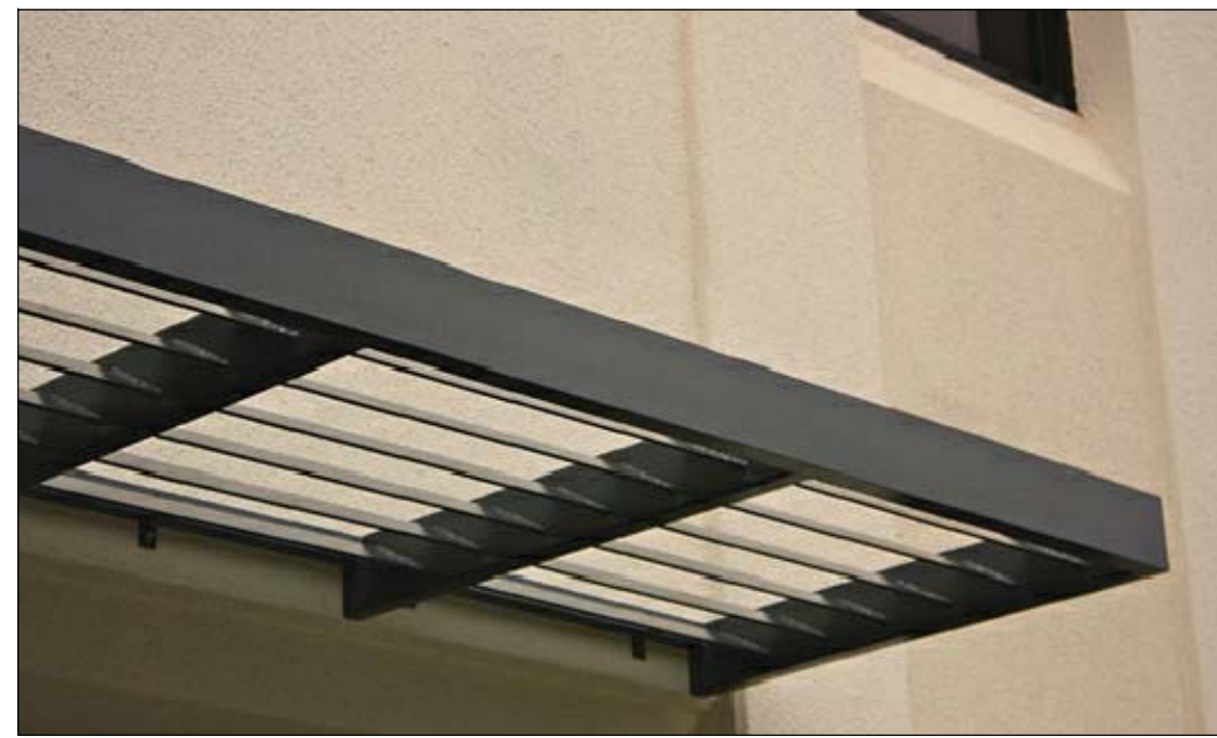
11 ANODIZED ALUMINUM SUNSCREENS ANCHORED TO FACE OF BUILDING
