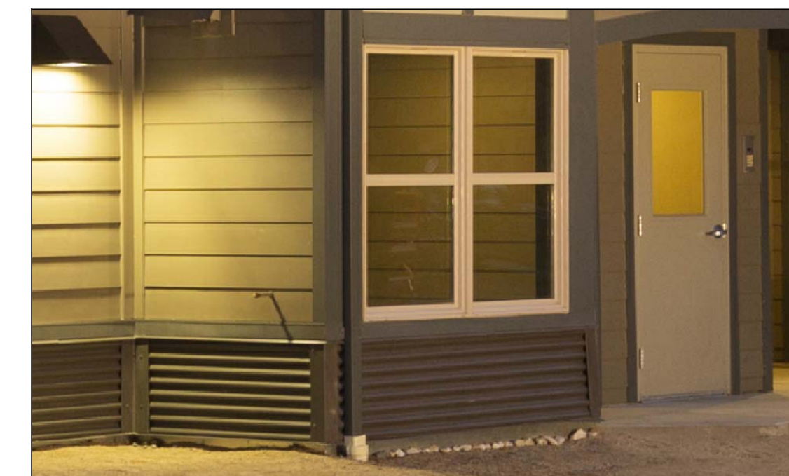
6 INSULATED, LOW-E VINYL WINDOWS
