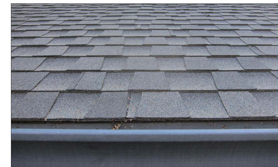
2 DIMENSIONAL COMPOSITION SHINGLE ROOFING - WEATHERED WOOD COLOR
