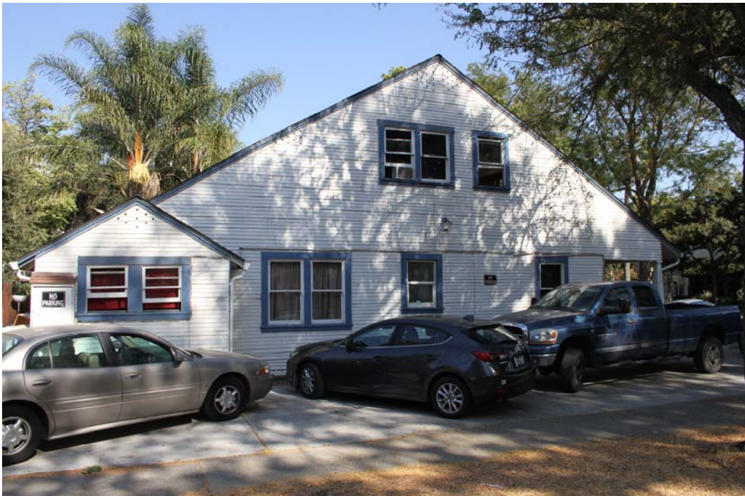
FIGURE 16: View looking east at the west elevation of 503 1st Street with the extended porch enclosure and addition of windows, including adding windows to what was once an attic on the second floor.
