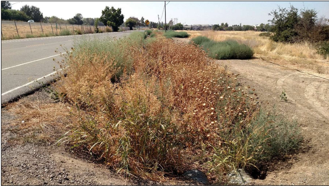
Non-jurisdictional roadside ditch (NJR-2), facing south – 16 August 2018
